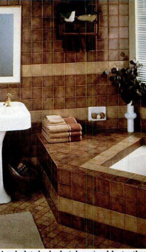
Angled tub deck (above) adds to the elegance that new tiles bring to this vintage bathroom. The deck, a simpler version of the one below, was scaled to minimize tile cutting. Deck's top (front) edge is exactly the width of two tiles plus grout lines. Deck height equals height of four tiles plus grout.
