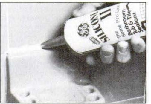
Multipurpose silicone permanently mounts ceramics onto bathroom tile (above left). Concrete-and-masonry ver-
