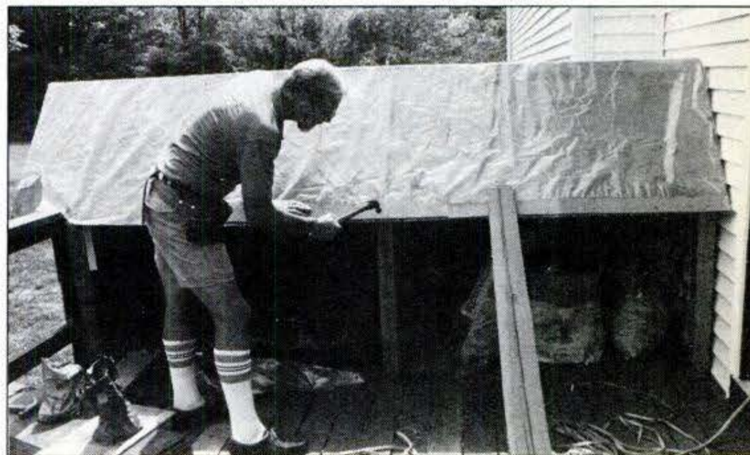
Begin by toenailing 2×4s in place (left). Nail rafters to both ends of the 2×6 ridge pole, and lift the beam into place (above). Nail remaining rafters in place (below left), and enclose with plywood. Tack paper in place before adding roofing and siding (below).
