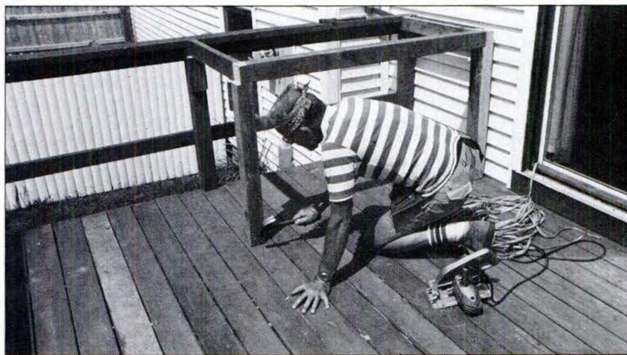
Begin by toenailing 2×4s in place (left). Nail rafters to both ends of the 2×6 ridge pole, and lift the beam into place (above). Nail remaining rafters in place (below left), and enclose with plywood. Tack paper in place before adding roofing and siding (below).
