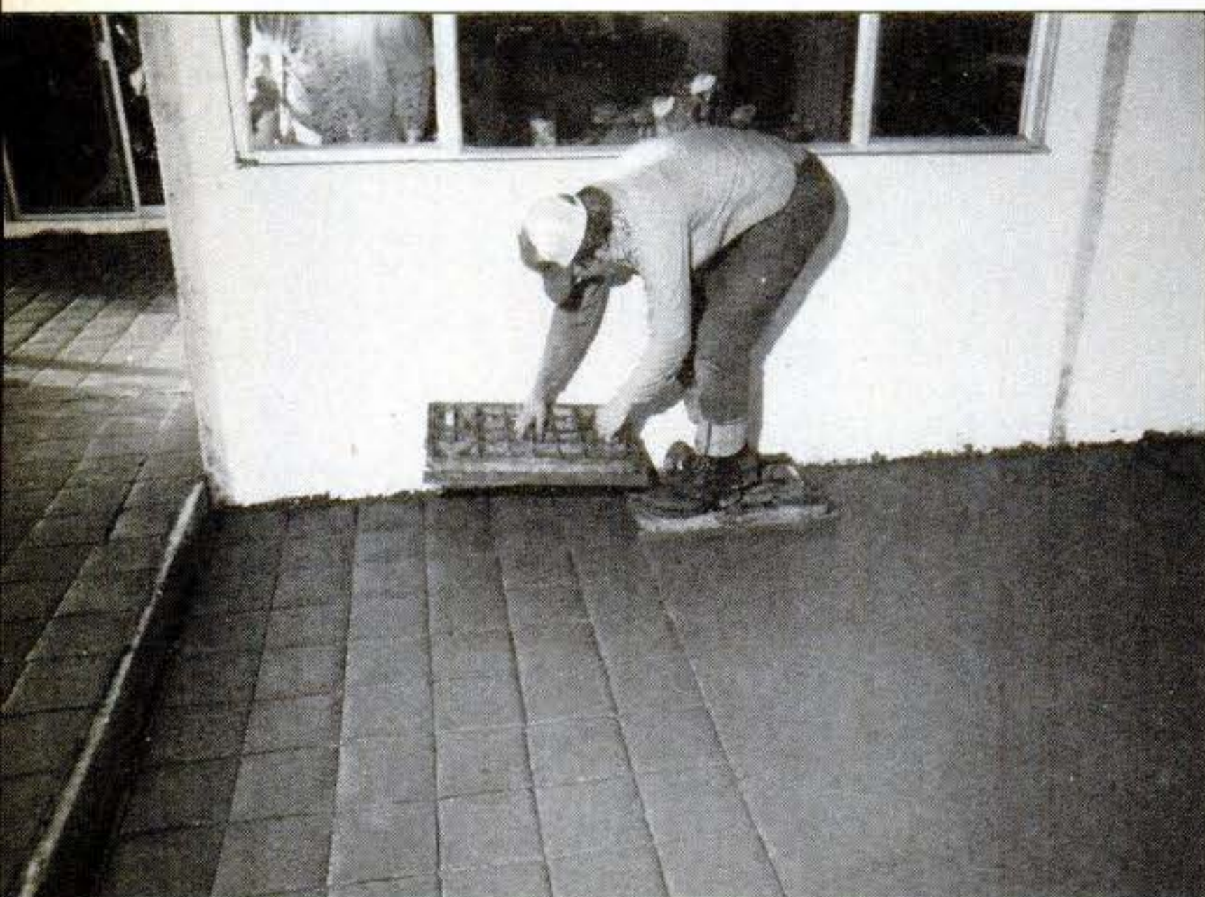
Author's crew tried two stamping methods. Here, stamper positions one pad while standing on another.
