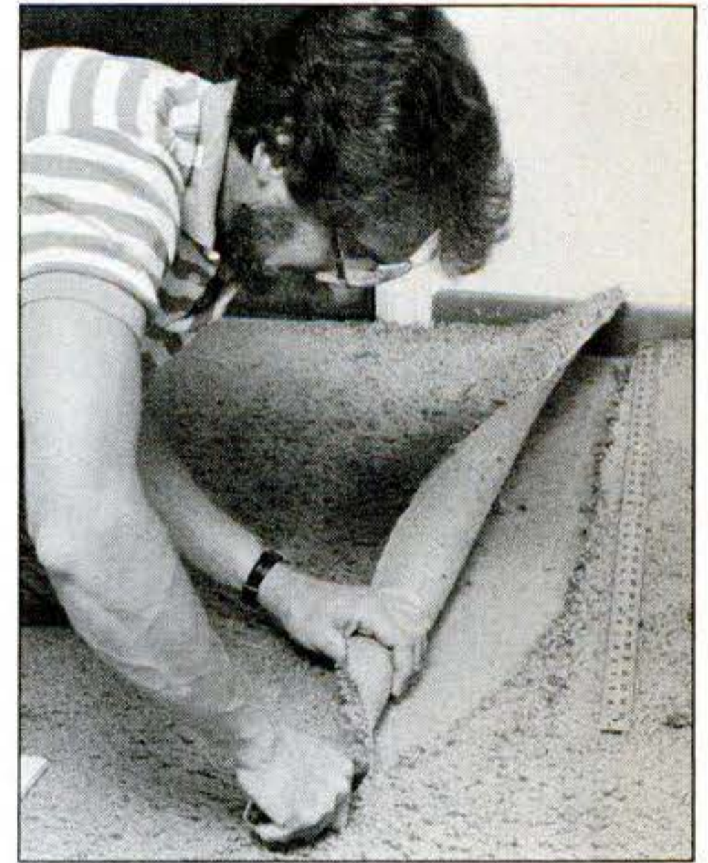
Heavy-duty knife is all that's needed to cut away the carpet and mat.
