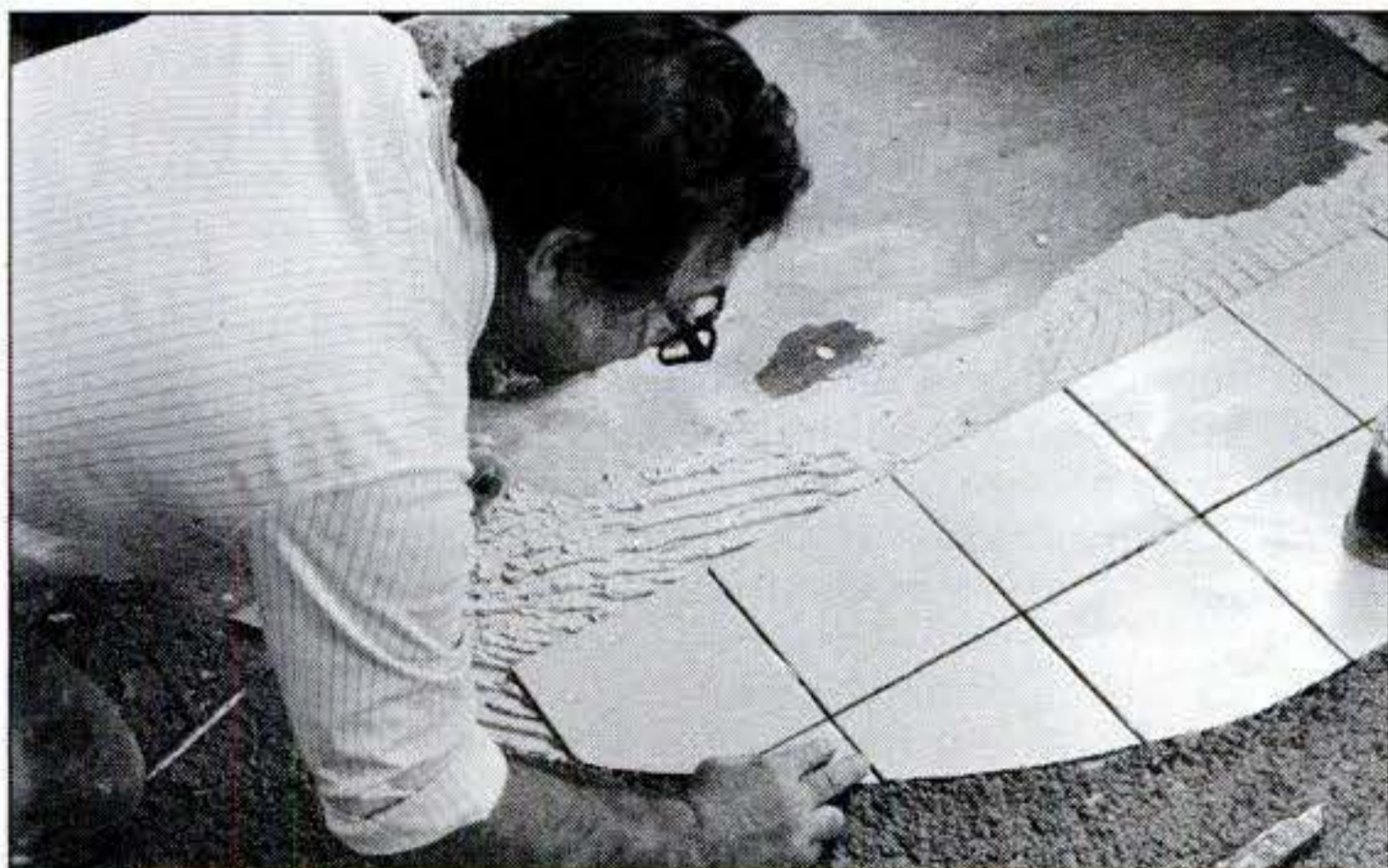
Lay the tiles out (above) to determine the grout lines and the number of tiles you'll have to cut to fit. Joint width should be roughly equal to the thickness of the tile. Cut
