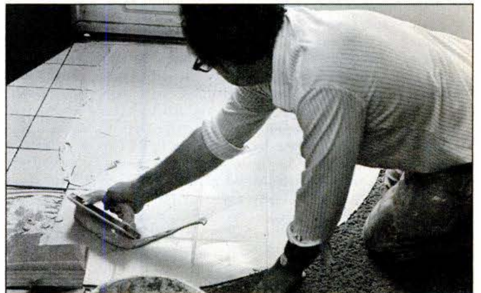
and fit the plywood form as shown in the photo (above right). Place tile down firmly (below left), and use a rubber-faced float to spread grout into joints (below right).
