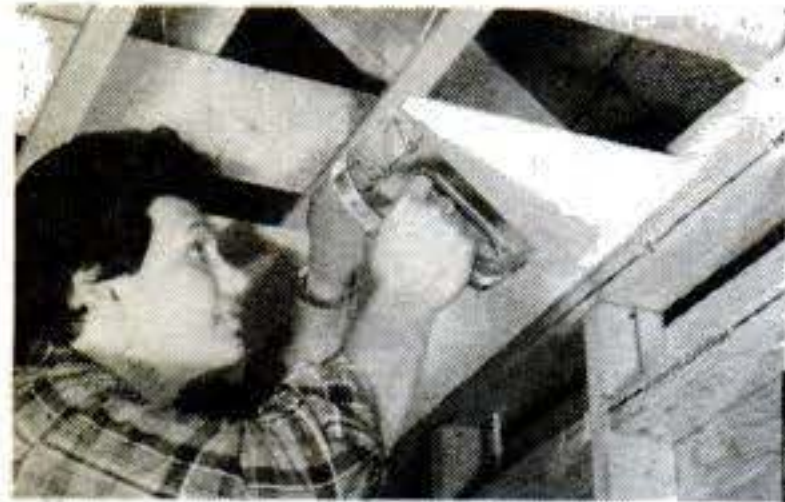
insulating an attic
