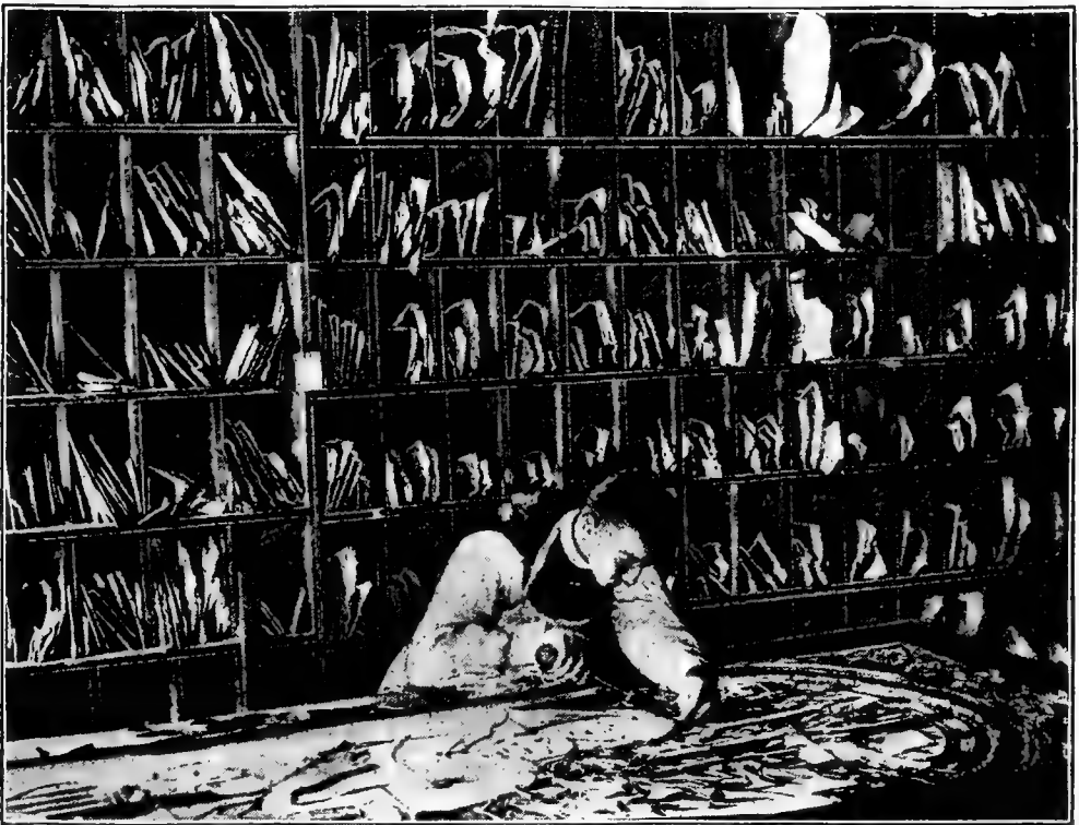
SOLDERING JOINTS OF LEAD LINES.
