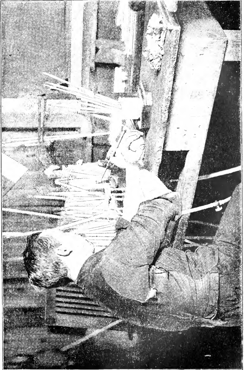
FIG. 4.—BLOWING THERMOMETER-BULBS.
