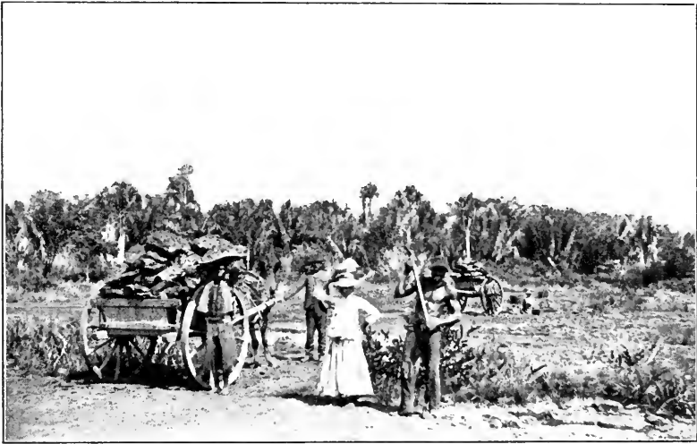
FIG. 2. DIGGING AND REMOVING PITCH FROM THE LAKE PRIOR TO 1890.
