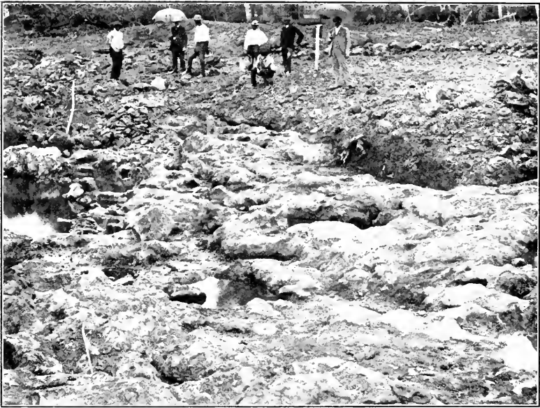
FIG. 5. A LOT OUTSIDE THE LAKE THAT HAS FILLED IN SIX MONTHS AFTER BEING EXCAVATED 20 FEET.
