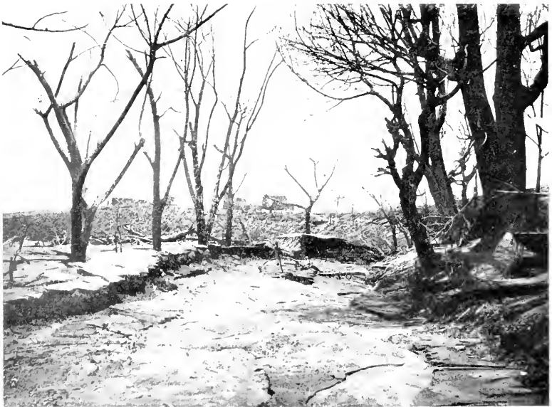
FIG. 13. ST. VINCENT: AVENUE FROM RICHMOND HOUSE TO THE SUGARWORKS, one mile from Chateau Belair. Just within the destruction belt showing the ruin of Richmond House. In location Richmond was the St. Pierre of St. Vincent.
