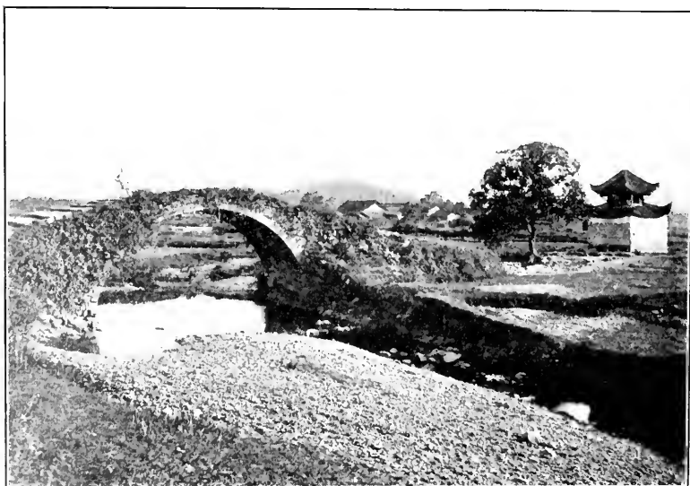
TEN LI BRIDGE PASSED BETWEEN KIUKIANG AND KULING.
