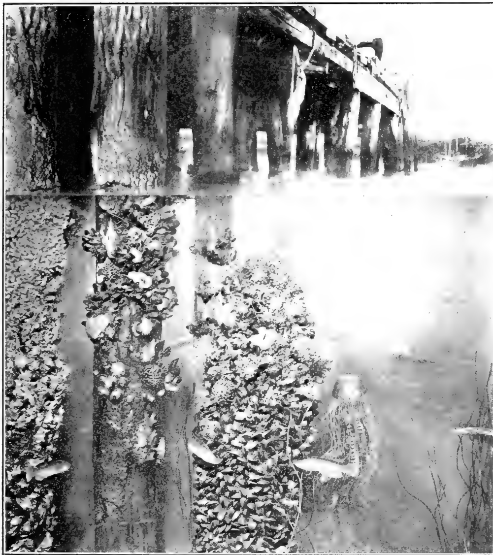
THE VINEYARD HAVEN WHARF PILE GROUP.
