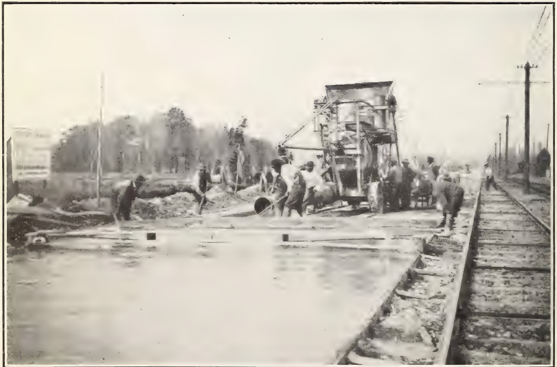
FIG. 2.—PLACING CONCRETE AND USING TEMPLATE.
