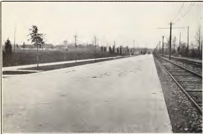
FIG. 2.—AFTER NEARLY TWO YEARS' SERVICE. EXPERIMENTAL CONCRETE ROAD, CHEVY CHASE, MD.
