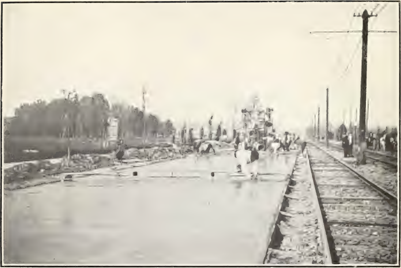
FIG. 1.—FINISHING THE SURFACE WITH A WOODEN FLOAT.
