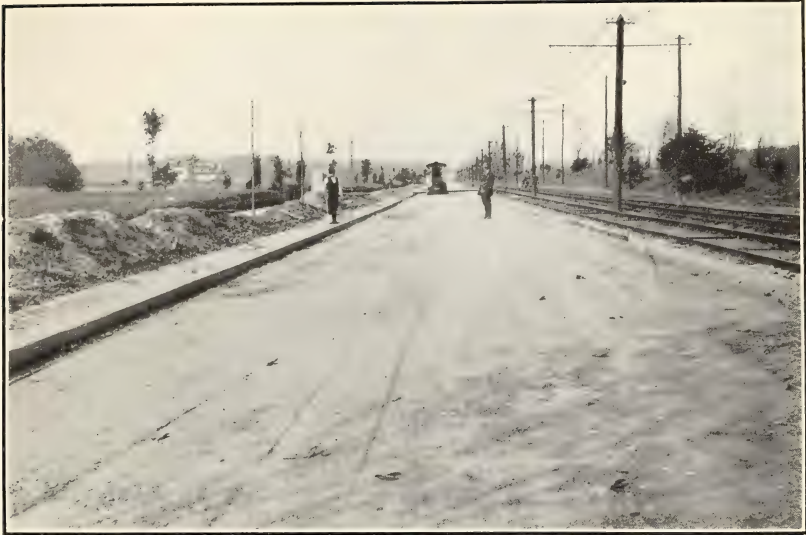
FIG. 1.—PREPARING SUBGRADE.
