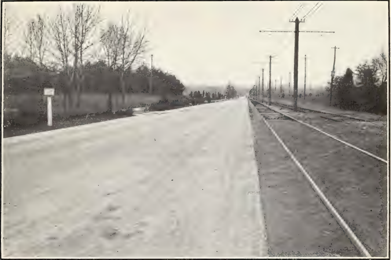
FIG. 1.—BITUMINOUS WEARING SURFACE IN FAIR CONDITION AFTER ABOUT ONE YEAR'S SERVICE.
