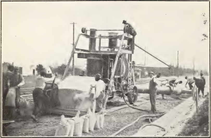
FIG. 1.—CHARGING CONCRETE MIXER.
