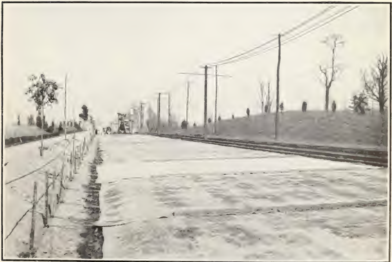
FIG. 2.—CANVAS COVERING IN PLACE.
