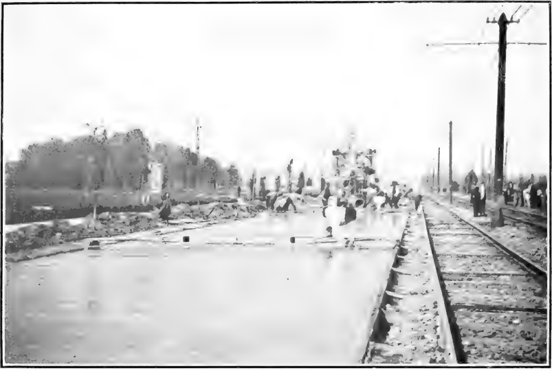
FIG. 1.—FINISHING THE SURFACE WITH A WOODEN FLOAT.
