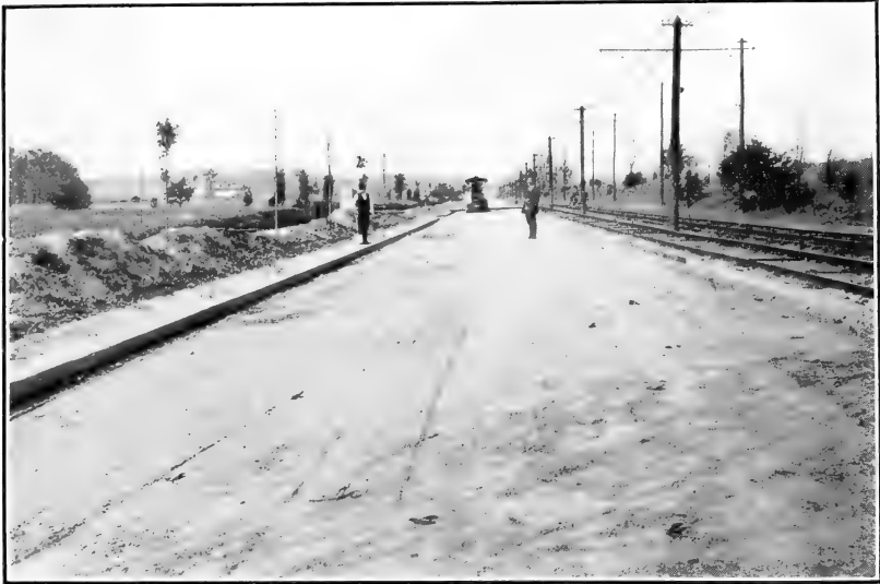
FIG. 1.—PREPARING SUBGRADE.
