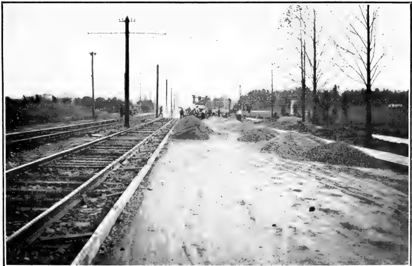
FIG. 2.—SAND AND GRAVEL PILED ON SUBGRADE READY FOR USE. EXPERIMENTAL CONCRETE ROAD, CHEVY CHASE, MD.
