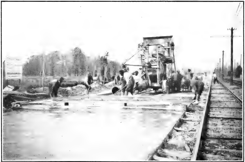
FIG. 2.—PLACING CONCRETE AND USING TEMPLATE.
