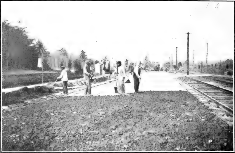
FIG. 1.—COVERING THE SURFACE WITH A LAYER OF EARTH AFTER CANVAS IS REMOVED.
