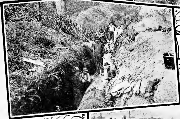
Riveting Pipe
