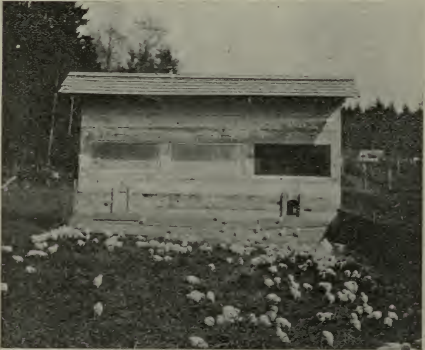
Colony brooder-house, 14 feet long and 10 deep; curtain-fronted. This house is built on skids and can be easily hauled by a team.
