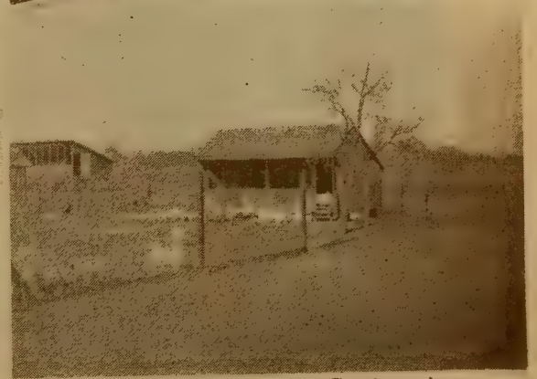
Fresh Air House for Cockerels
