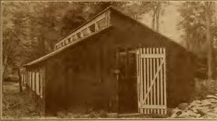
COCKEREL AND CONDITIONING HOUSE
