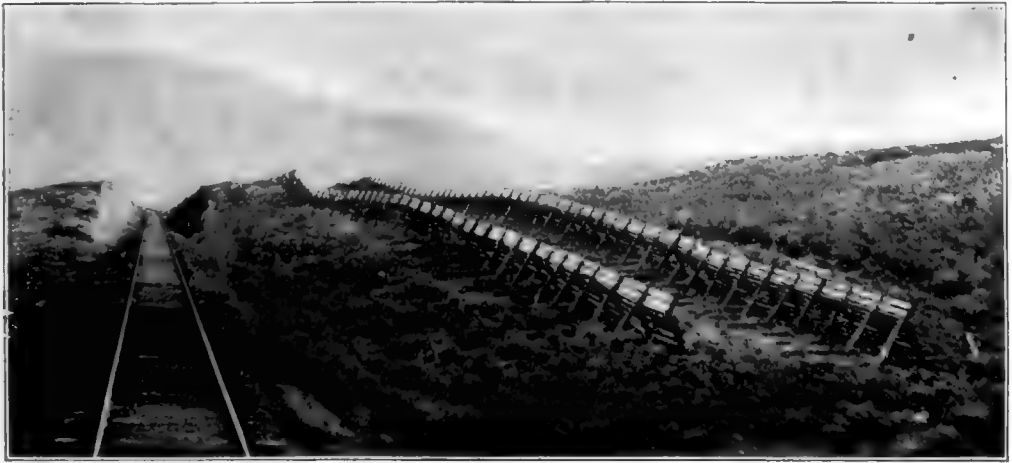
DOUBLE LINE OF SNOW FENCES ON RIO GRANDE WESTERN RAILWAY, UTAH.
