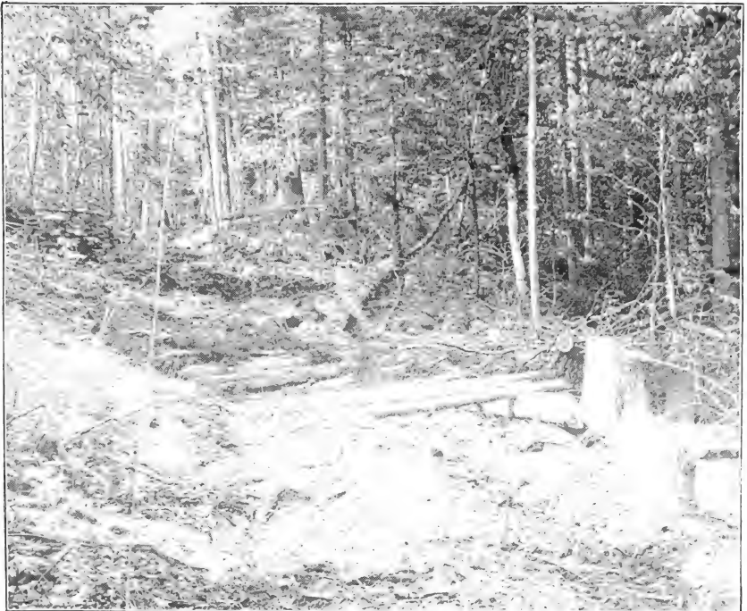
FIG. 2.—SMALL SPRUCE USED IN LEVELING A LUMBER ROAD. WHITNEY PRESERVE.
