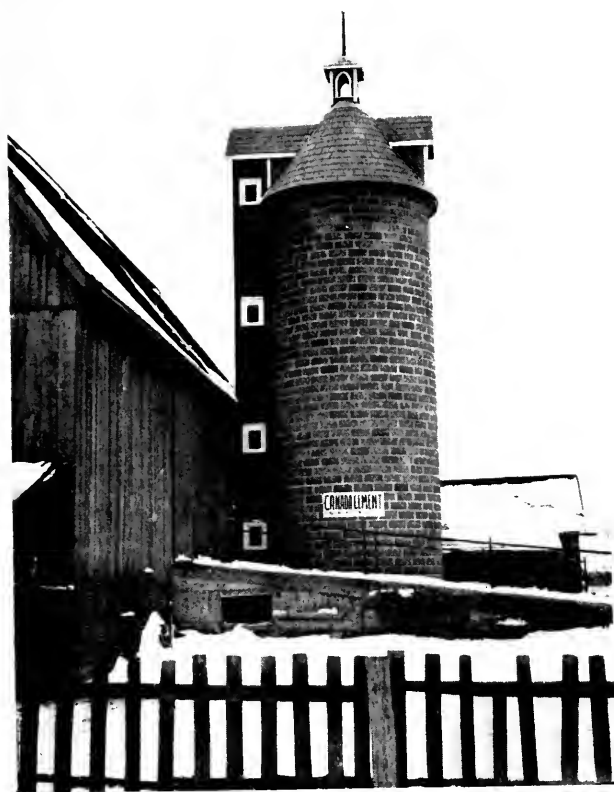
Fig. 5.—The tall, round silo is best. This one is built with concrete blocks
