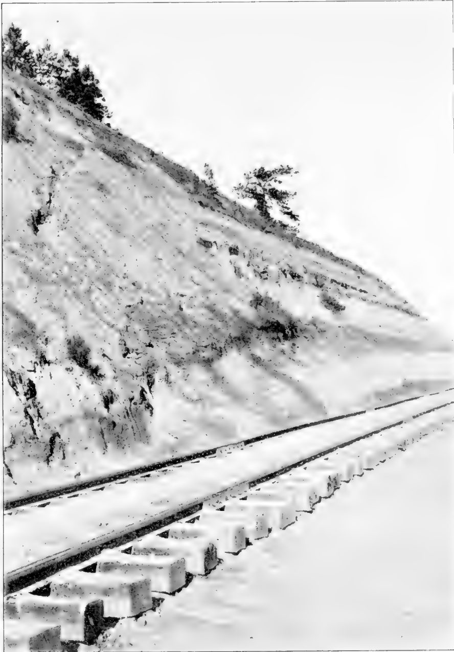
CUT SOUTH OF STATION, COLUMBIA, LA.
