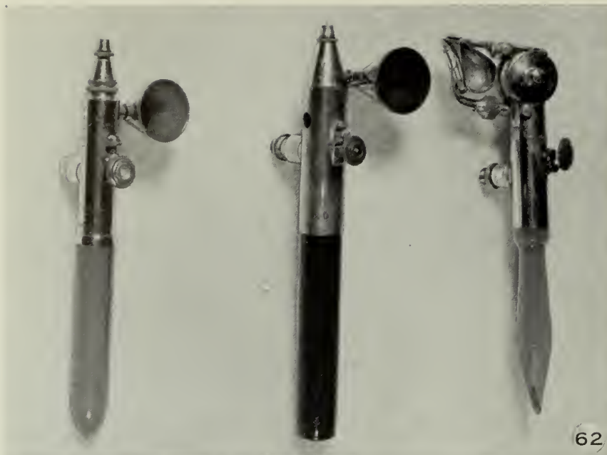
Figure 62 Airbrushes. Left, Wold Center, Thayer and Chandler. Right, Paasche.
