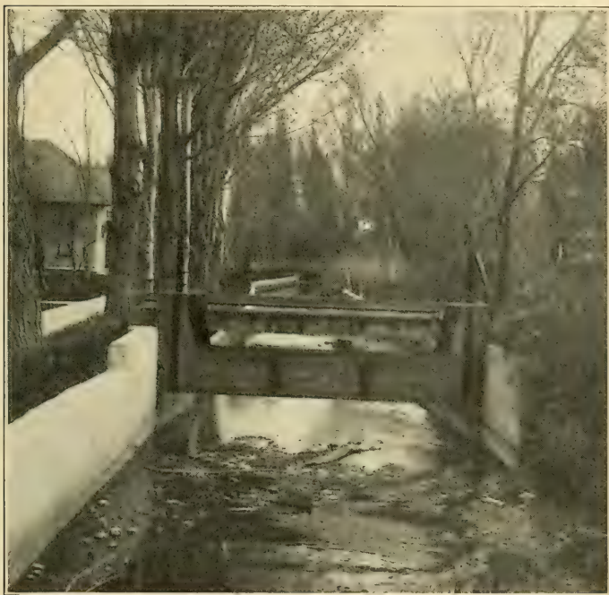
FIG. 23. — A good type of weir for measuring irrigation water.
