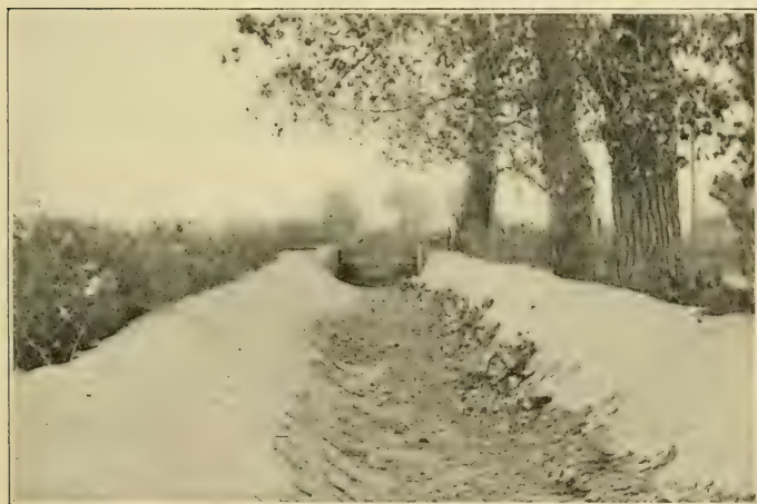
FIG. 21. — Cement lining prevents seepage.
