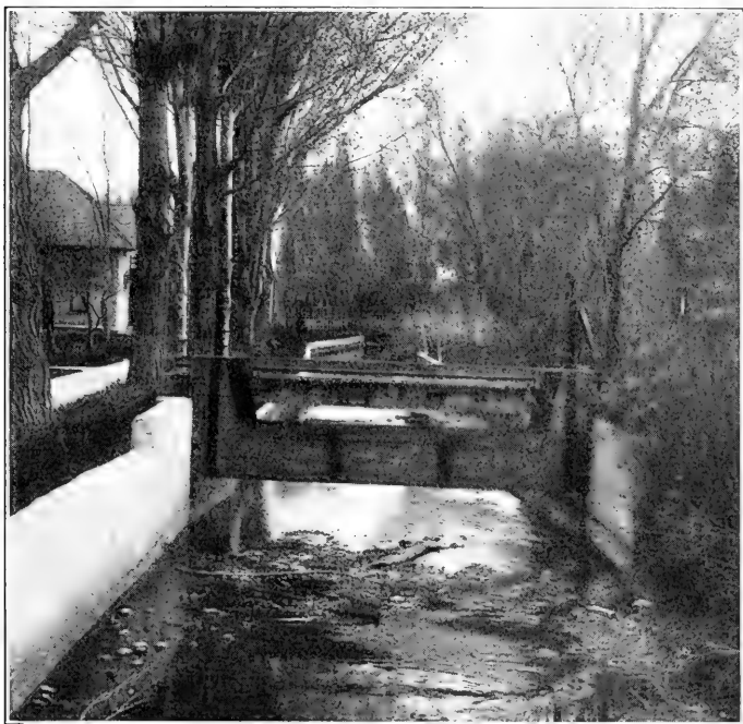
FIG. 23. — A good type of weir for measuring irrigation water.
