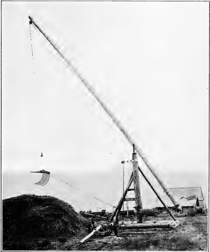
FIG. 71. — A convenient device for stacking hay.
