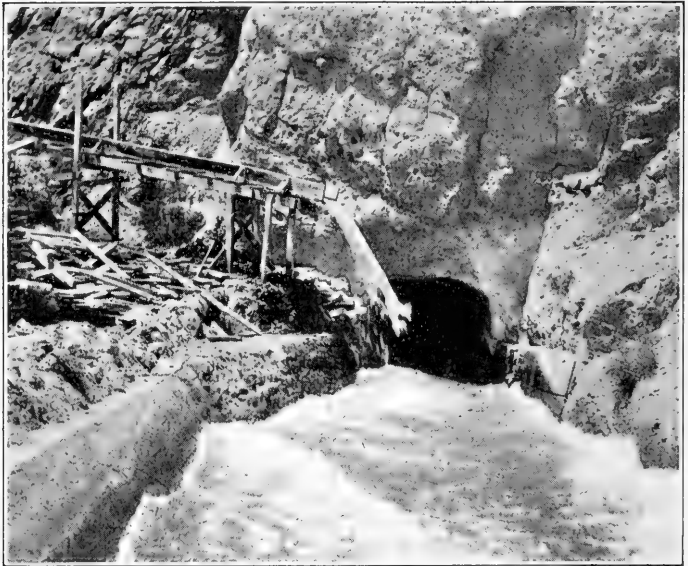
FIG. 22. — Water diverted from reservoir through tunnel in rock.
