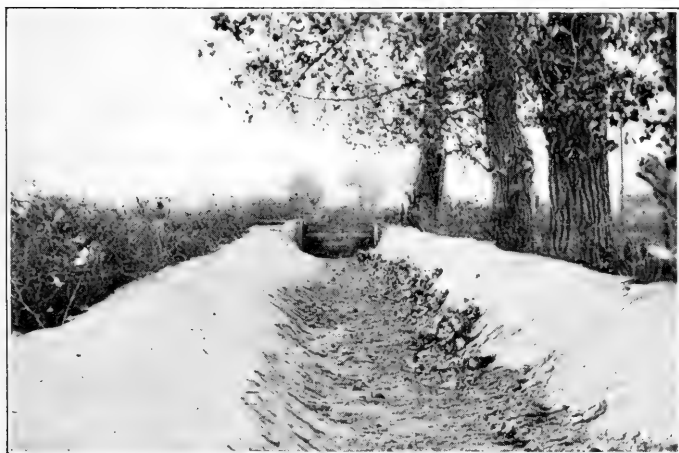
FIG. 21. — Cement lining prevents seepage.
