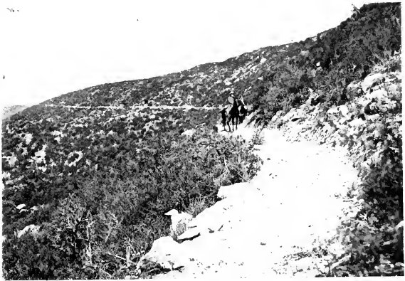
FIG. 59. A Mountain Trail Built for Fire Patrol. Angeles National Forest, California.
