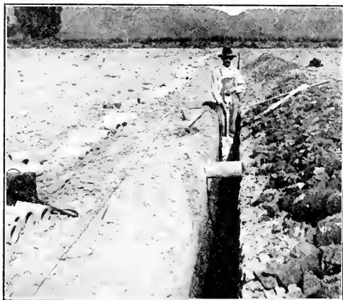
FIG. 81. Construction of a ditch for tile drains.
