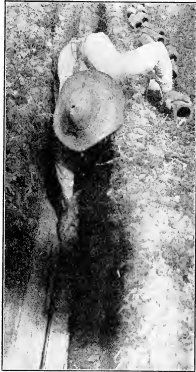
FIG. 83. Laying double-sole drain-tile by hand.
