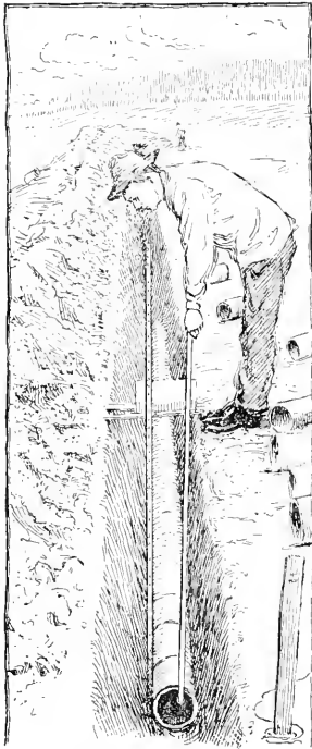
FIG. 82. Laying tile in the bottom of ditch by use of the tile hook. Shows arrangement of tile preparatory to filling the ditch.
