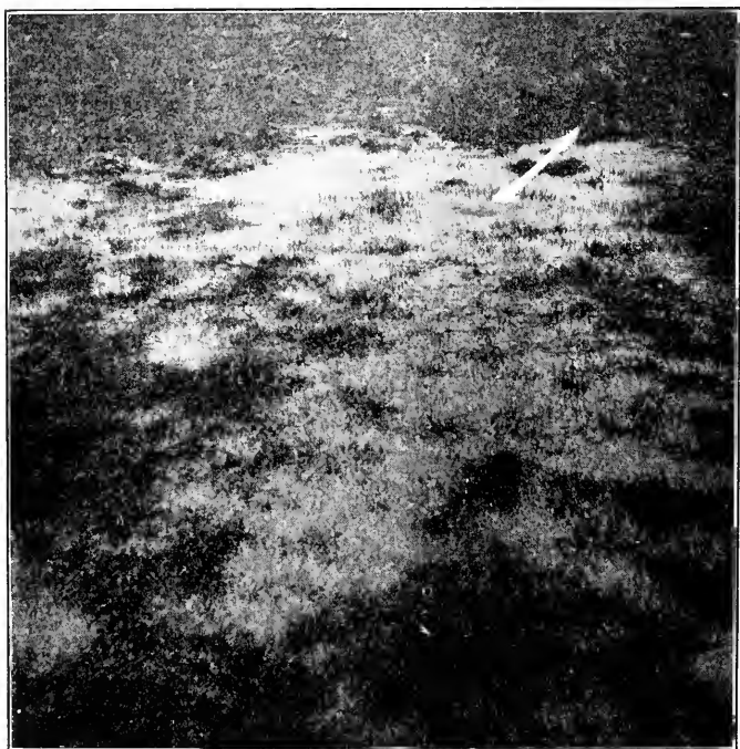
FIG. 94. Water forced to the surface by the closure of the outlet of a tile drain.
