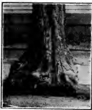
FIG. 302—MUTILATED TO LAY A CURB
