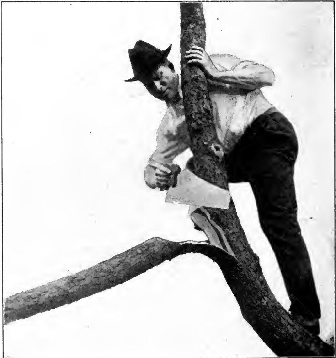
FIG. 89—WRONG WAY TO CUT OFF BIG LIMB
