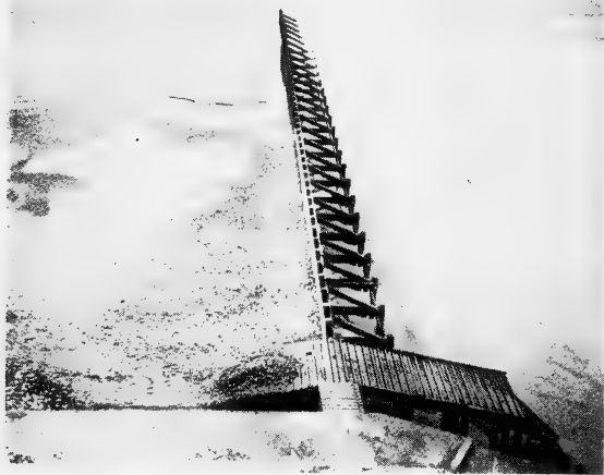
B.—GROYNE AT OVERSTRAND, NORFOLK. The shingle tends to move southwards and so is heaped on the northern (left) side of the groyne.
