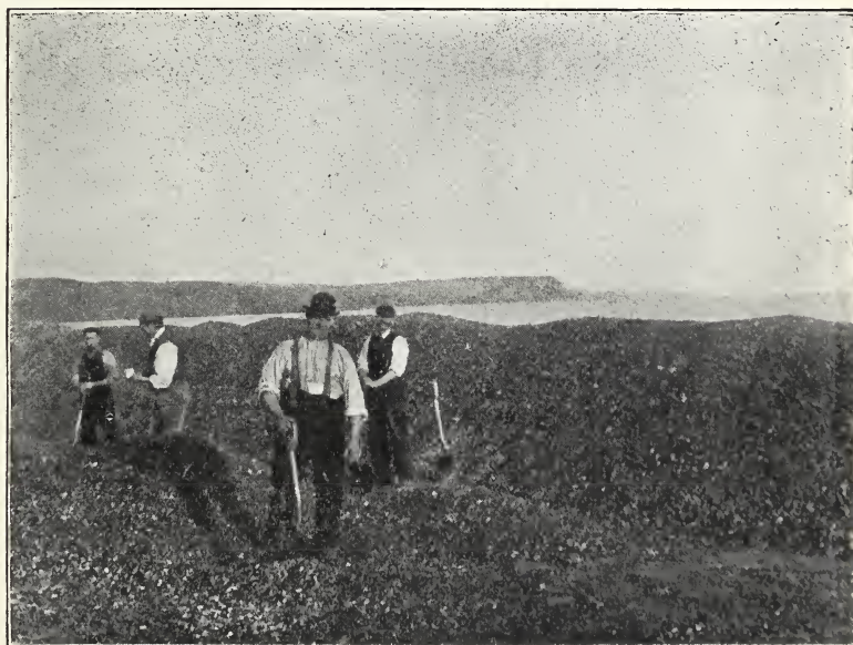
4.—MEN CLEARING SHINGLE FROM ROAD (NEARER COASTGUARD STATION THAN 3). SHINGLE 3FT. DEEP OR MORE OVER ROAD.
