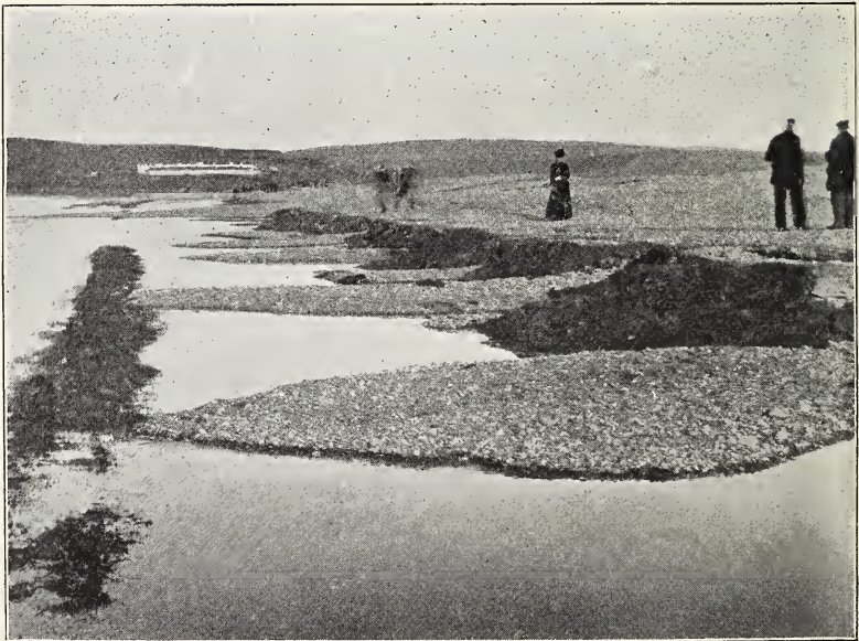
2.—VIEW OF LODMOOR SIDE OF BEACH, SHEWING DAMAGE TO ROAD AND SHINGLE PROMONTORIES WASHED INTO LODMOOR.
