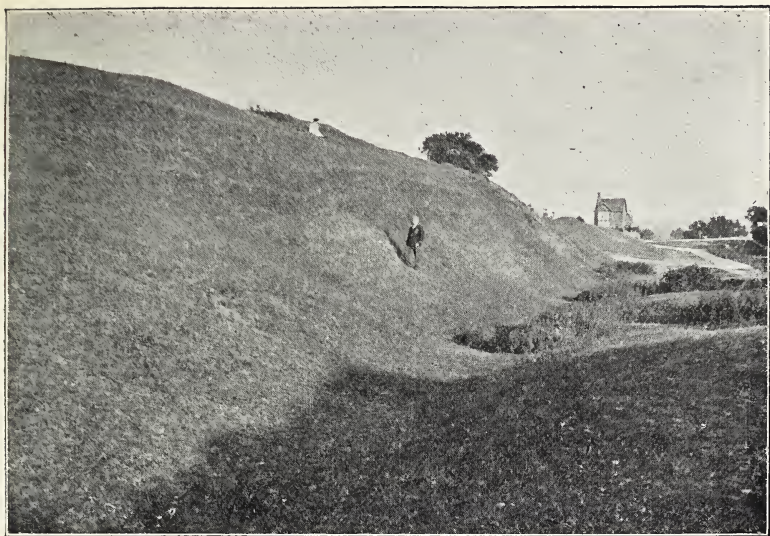
WEST WALL OF WAREHAM AND DITCH, TAKEN FROM BLOODY BANK. THE PORTION OF DITCH REMAINING IS 51 FEET WIDE; THE DEPTH VARYING FROM 28 TO 34 FEET.
