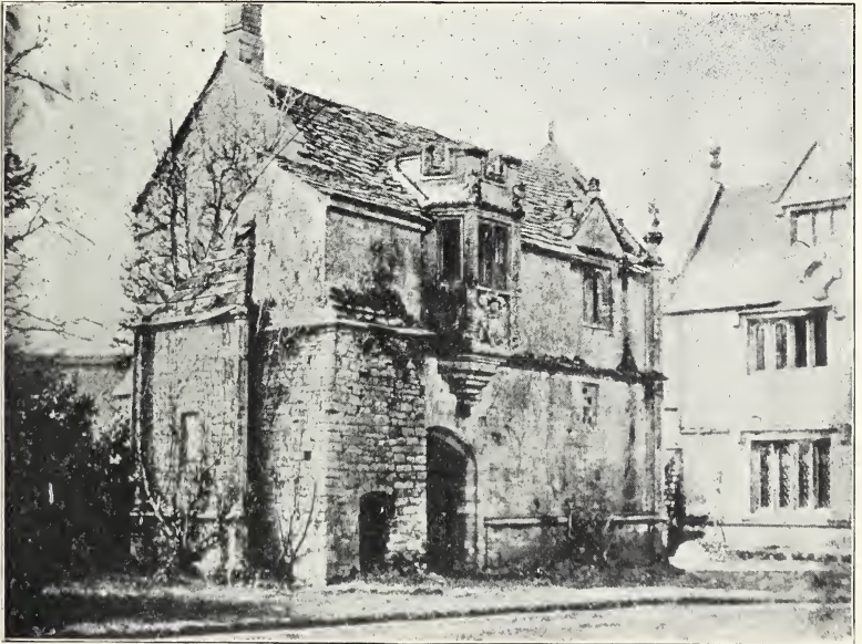
GATEHOUSE AT ATHELHAMPTON FROM A PHOTOGRAPH TAKEN THE DAY BEFORE IT WAS PULLED DOWN IN 1862.
