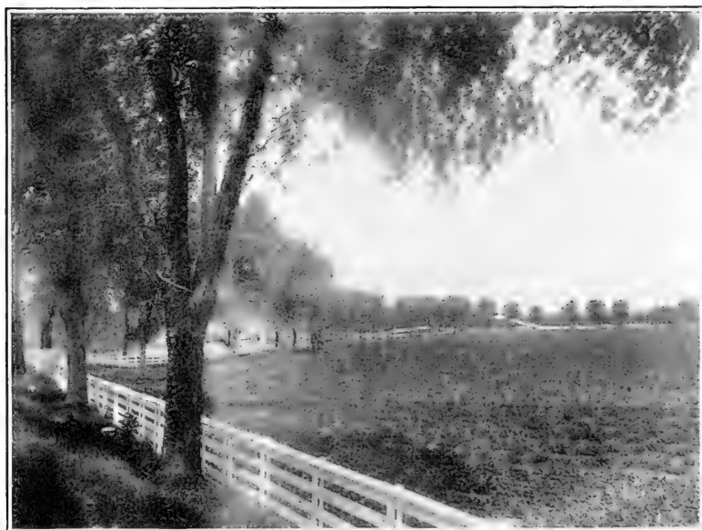
Field to be irrigated and fertilized by effluent from Septic Tank, as seen from main drive.
