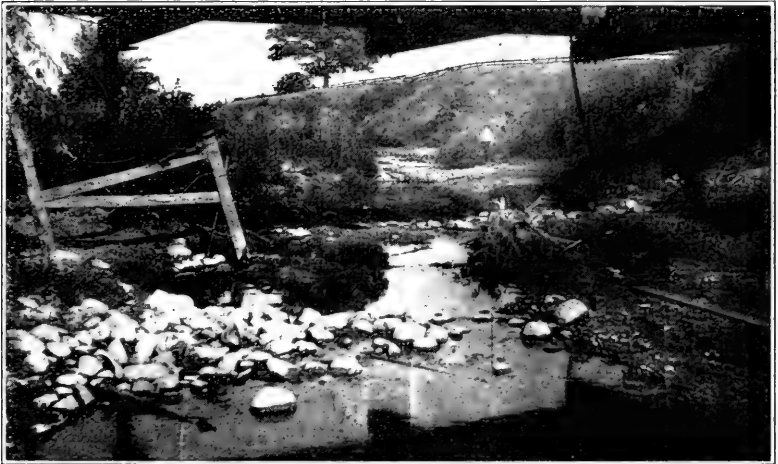
Fig. 7. View up the channel of the outlet at the greater dam. The depth of the valley is shown by the altitude of the right abutment in the background. The evidence of the ascending erosion line is in the foreground.
