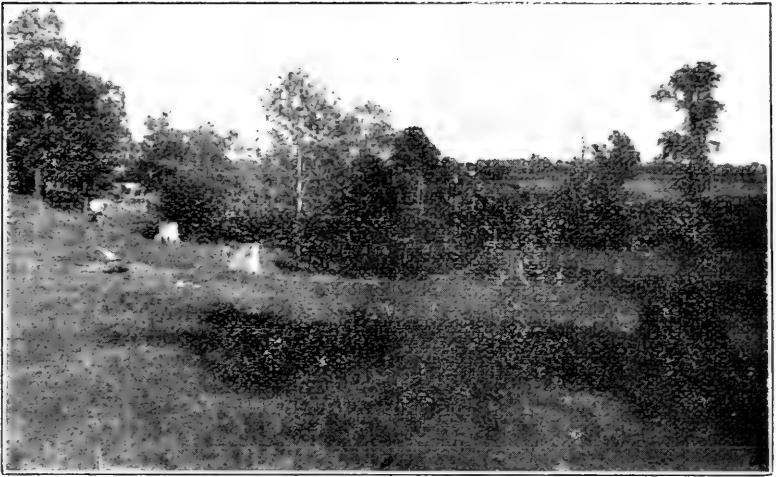
Fig. 6. View across the valley from the left abutment of the lower or greater dam. The width of the valley is here about 165 feet, with the earth walls rising abruptly 22 feet on either side. The soil is a glacial deposit, sand predominating.
