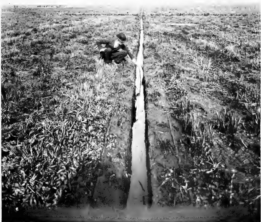
10" WIDE DITCH CLEANED BY MACHINE
