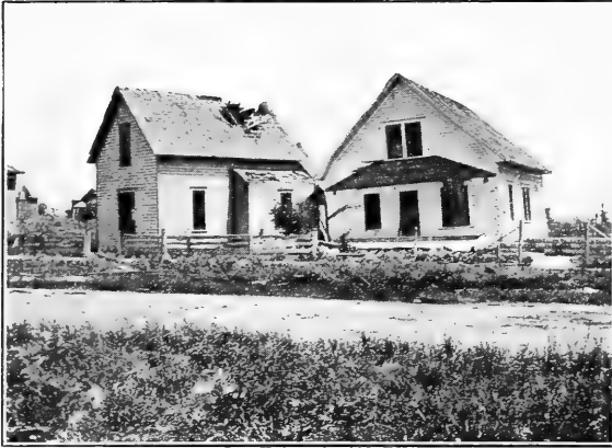
FIG. 13. House moved from foundation. Watertown, S. D., June 23, 1914.
