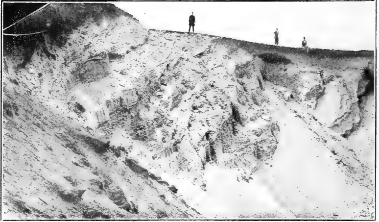
Shawnee Mound. Excavation in North Side showing Material and Arrangement.
