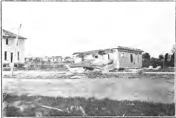
FIG. 12. House moved from foundation. Watertown, S. D., June 23, 1914.
