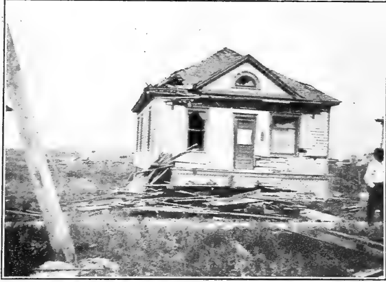
FIG. 15. The tornado passed to the left of this house moving toward the reader. The porch was torn away and deposited in the rear of the house. Watertown, S. D., June 23, 1914.
