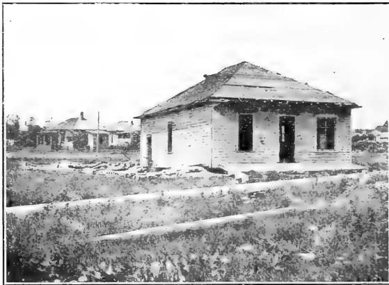
FIG. 16. House moved from its foundation. Shingles stripped from roof. Tornado passed to the right of it. Watertown, S. D., June 23, 1914.
