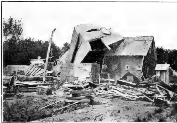
FIG. 14. Effects of tornado, Watertown, S. D., June 23, 1914.
