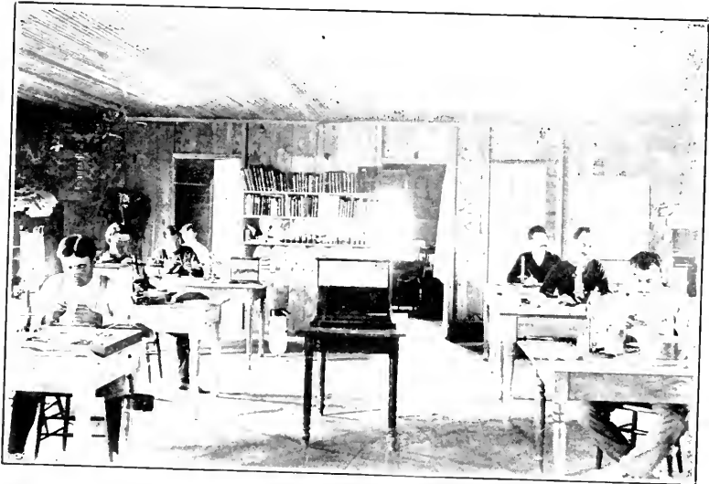
Upper Floor, Lake Laboratory.
