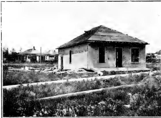
FIG. 16. House moved from its foundation. Shingles stripped from roof. Tornado passed to the right of it. Watertown, S. D., June 23, 1914.
