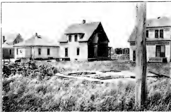
FIG. 4. House with end blown outward.
