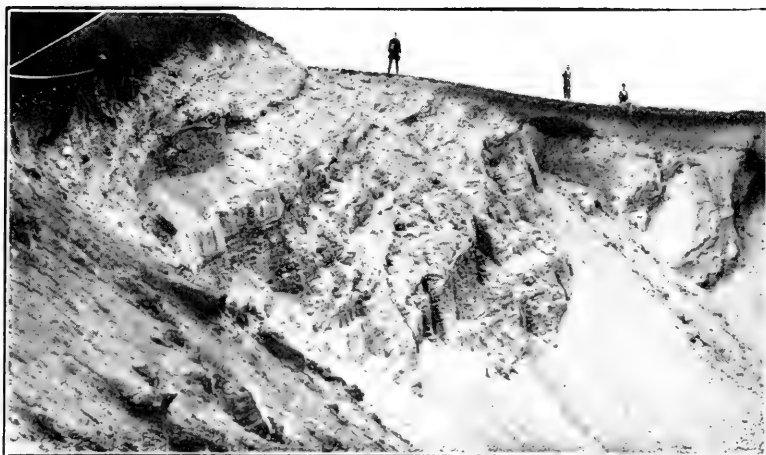
Shawnee Mound. Excavation in North Side showing Material and Arrangement.
