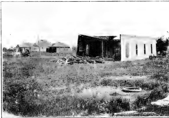
FIG. 5. House in east Watertown, S. D., showing explosive effect of air during passage of tornado.
