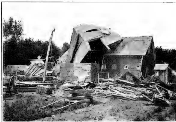
FIG. 14. Effects of tornado, Watertown, S. D., June 23, 1914.
