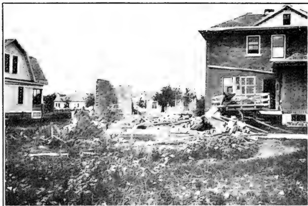
FIG. 9. Collapse of hollow tile structure. Watertown, S. D., June 23, 1911.
