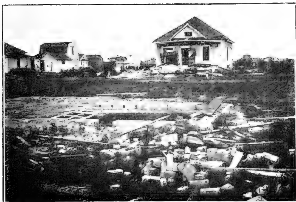
Fig. 10. The house from the foundation in the foreground was carried bodily across the street and then dropped to the earth and broken to bits. Wreckage may be seen in front of cottage on the right.
