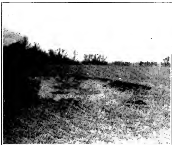
FIG. 23.—A washout made by the flood of 1913 in a cultivated field. The dark areas in the bottom of the excavation mark the extent to which revegetation had been carried on in two years. Location C, figure 16.
