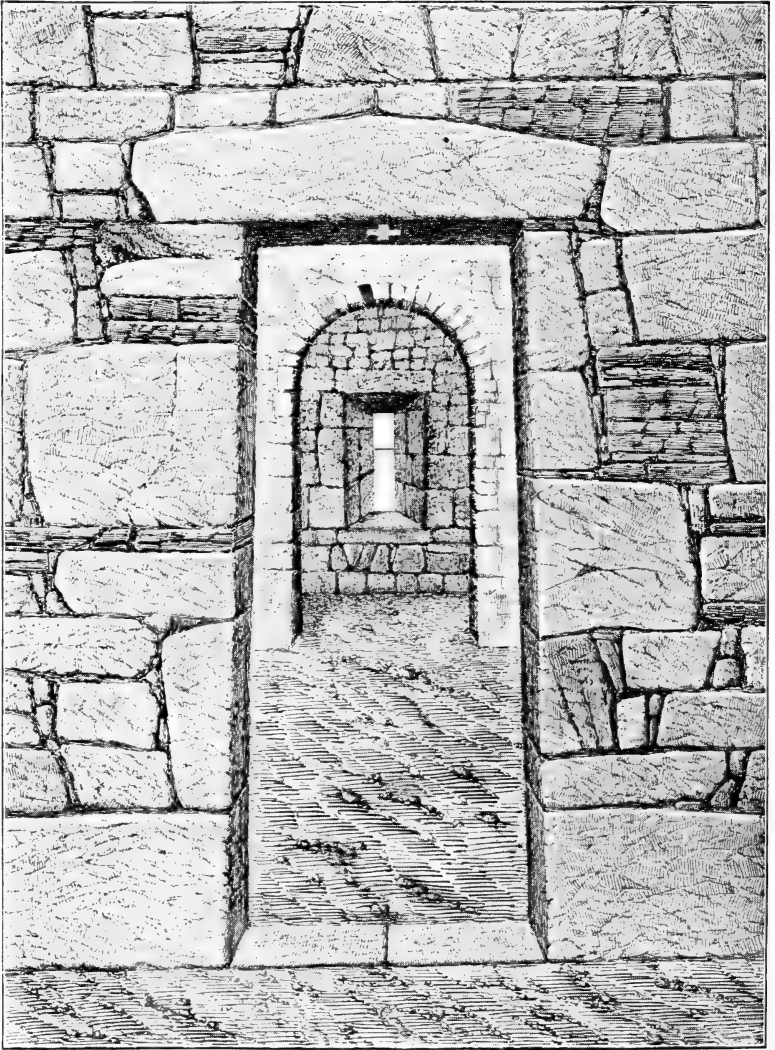
WESTERN DOORWAY OF KILLINEY CHURCH,
