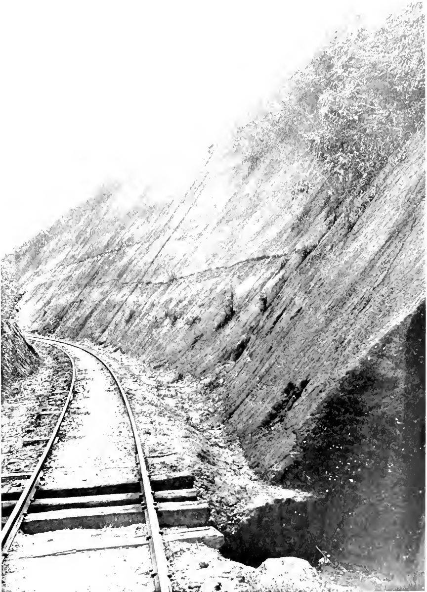
Deep cut near Bittencourt on the Alagôas railway, exposing sedimentary rocks of the Alagoas Group.
