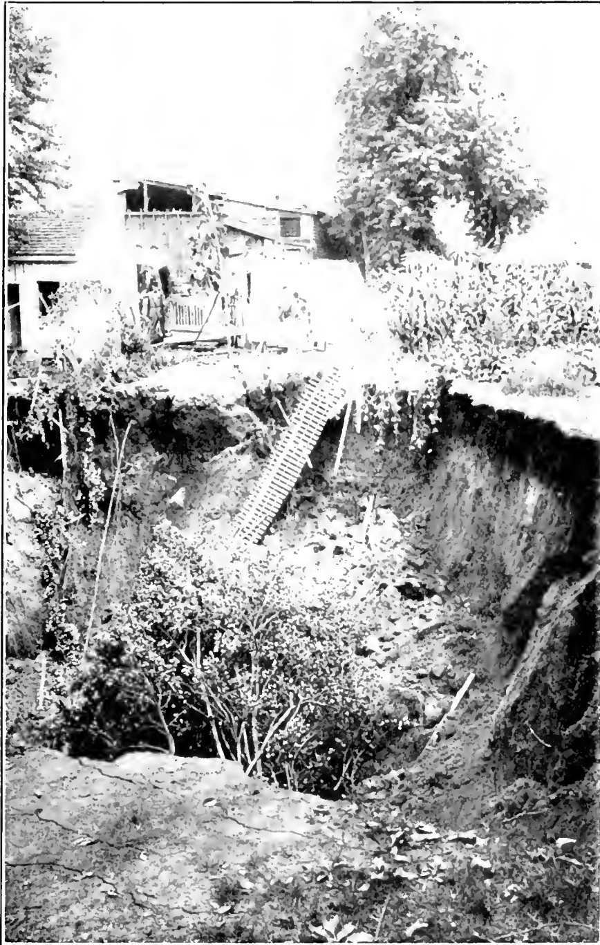
View showing an early stage of "cave-in" No. 3.
