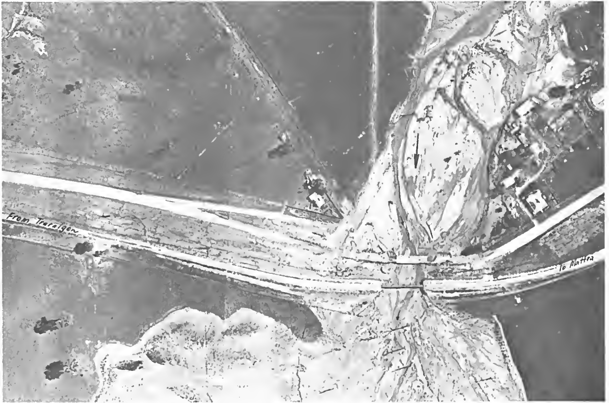
Fig. 5—Aerial photograph of the main road and rail bridges taken just after the 1952 floods, showing sand splays. (Source: Victorian Railways).
