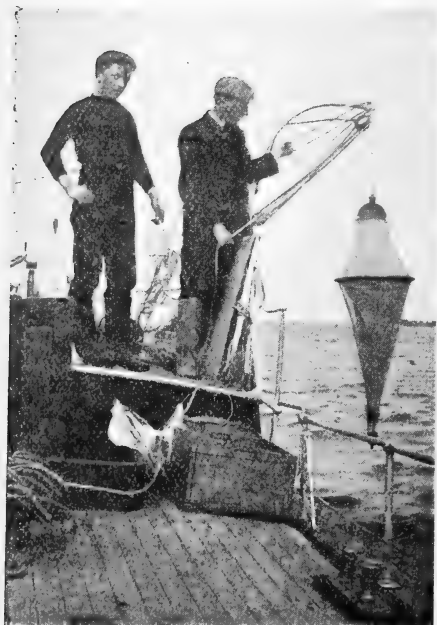
FIG. 7.—Closing Petersen-Hensen Net going down open.
