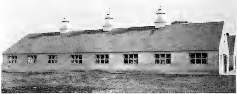
FIG. 85.—A well-lighted dairy barn. Note that top sash of windows fall inward to aid in ventilation. Owned by H. P. Hood and Sons, Boston. (Courtesy of James Mfg. Co.)
