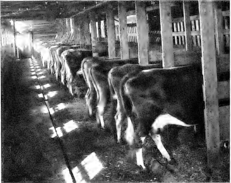
FIG. 92.—These cows keep themselves clean by stepping forward to lie down in front of the 2 x 4-inch stringer which holds the bedding in place. Note the broad shallow gutter, safe and easy to clean. (Owned by C. C. Graves, Maryville, Mo.)
