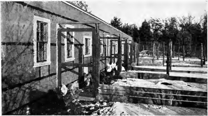
FIG. 64.—Antiquated type of poultry house, with no muslin in windows. Glass prevents ventilation and holds the moisture.
