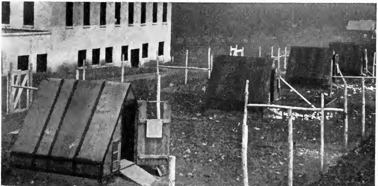
FIG. 168.—Portable gasoline brooder houses. A, Working plans; B, brooders in actual operation.
