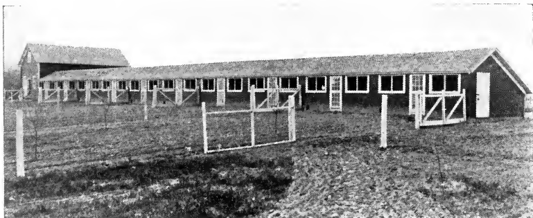
FIG. 89.—Laying house with two-thirds span roof. A neat house. The cost is greater and the front lower than with the shed roof.
