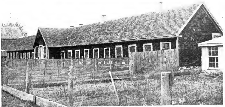
FIG. 163.—Three different types of long brooder houses. A , Feed house and boiler room in centre. The high fences make it possible to keep adult birds in the runs when they are not used for chicks. B , Wide "half-monitor" type of roof, allowing a centre walk and brooder pens on each side. C , House with gable roof and automatic ventilation.
