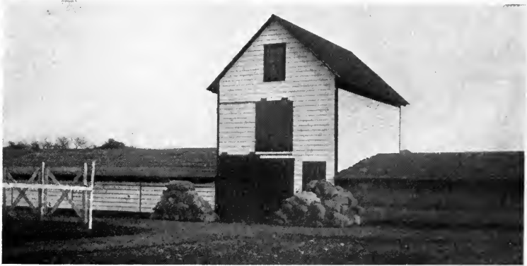
FIG. 118.—Poultry feed house centrally located, with long laying house on either side. The upper floor is used for storage of hay and grain, and the lower floor for mixing and weighing.
