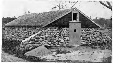
FIG. 19.—Incubator cellar in the South Shore district, Mass., showing economical construction with field stones laid in mortar. (Photo by E. O. Damon, owner.)
