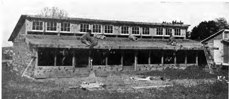
FIG. 91b.—Half-monitor type of laying house: Under construction.
