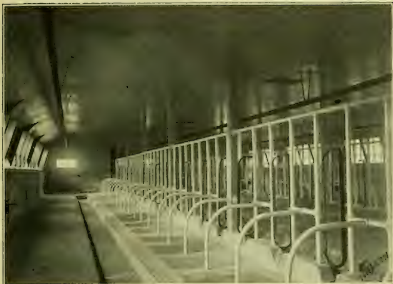
Interior view of a modern, sanitary dairy barn where certified milk is produced. Notice the cement floors and the boards placed on the cement for the cows to lie on.
