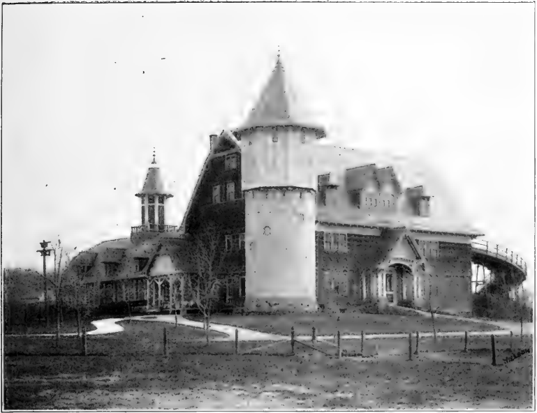
Dairy barn on the Wisconsin Experiment grounds, Madison, showing that art and utility may be combined with little additional expense. Note the artistic silo in the foreground, above which is placed a large water tank. To the left is seen the ventilating tower used in supplying the cow barn underneath with pure, wholesome air.
