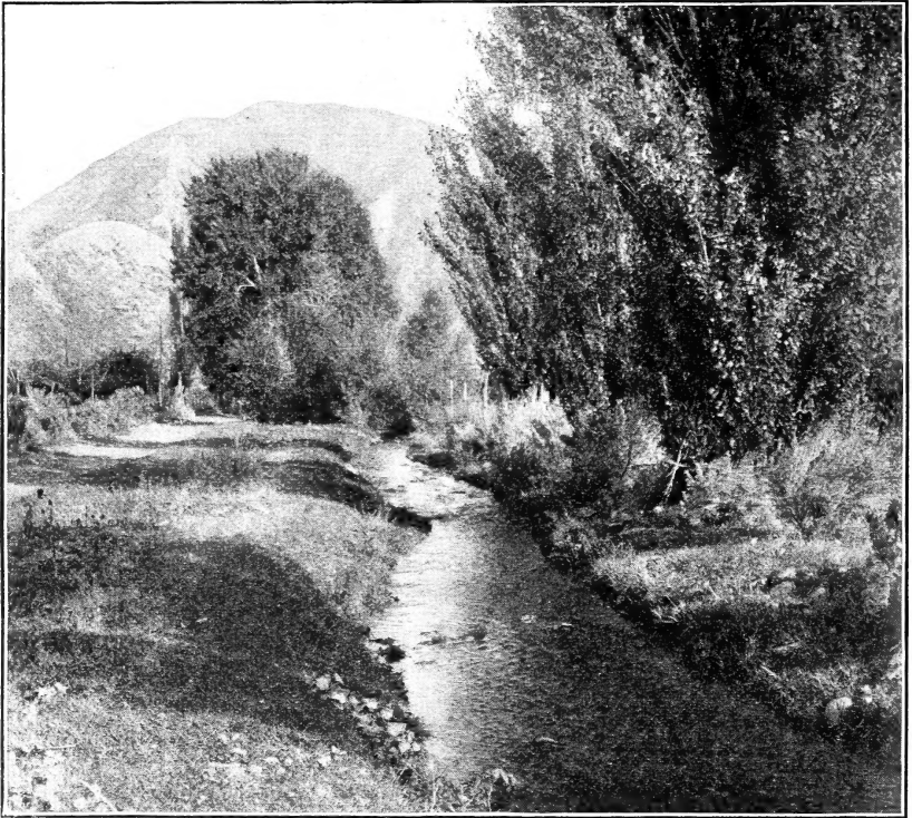
FIG. 3.—A wide irrigation ditch, entailing much waste of water.
