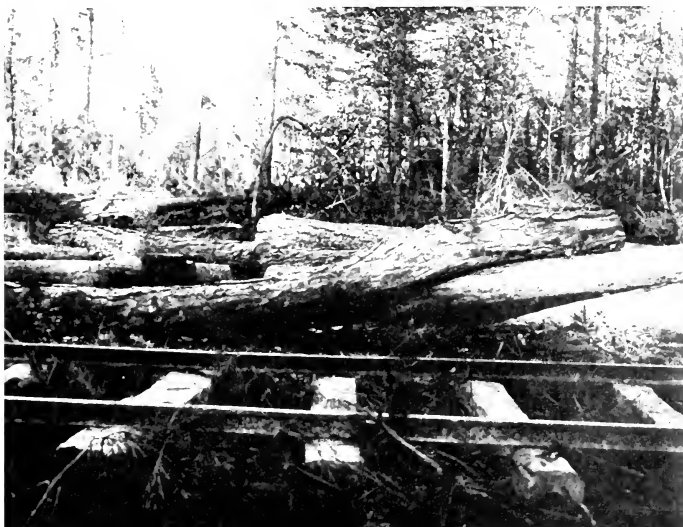
FIG. 2—VERY CROOKED LOG READY FOR LOADING
