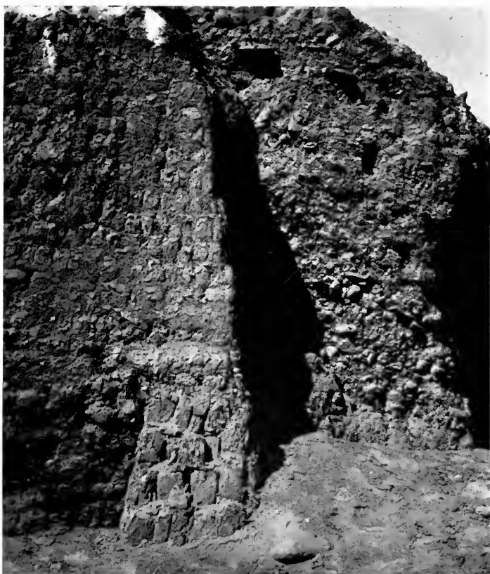
FIG. 5. Mud bricks alternating with sherds and rubbish at T and U in pyramid 16.
