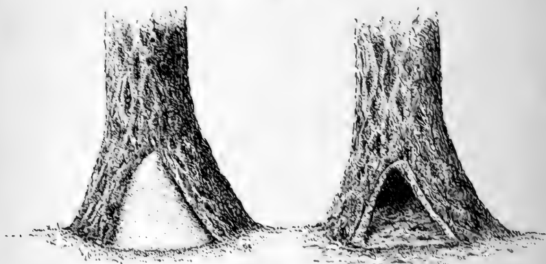
123. The cavity cleaned on the right; filled on the left.
