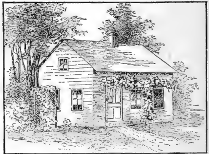
354. Vines about a building.
