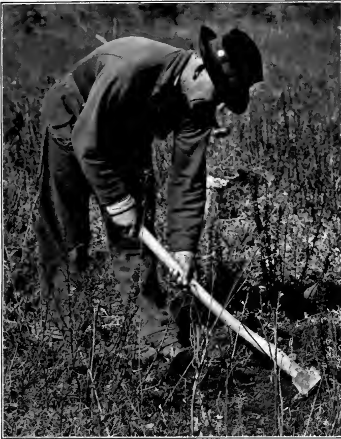
REMOVING TURF AND DIGGING HOLE
