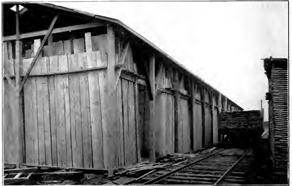
DRYING MAPLE LUMBER BY END-STACKING
