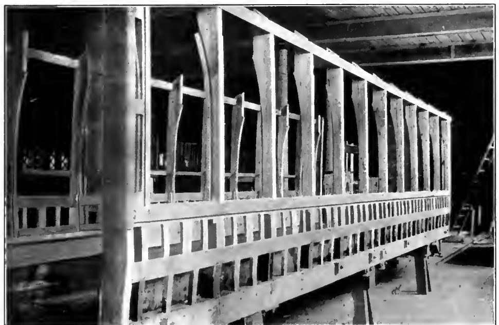
STREET CAR CONSTRUCTION
