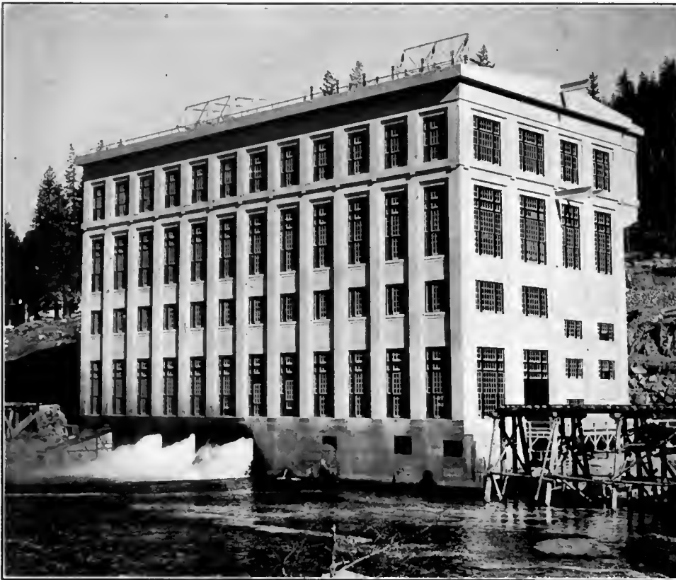
PLANT NO. 1 OF THE PACIFIC LIGHT AND POWER CORPORATION
