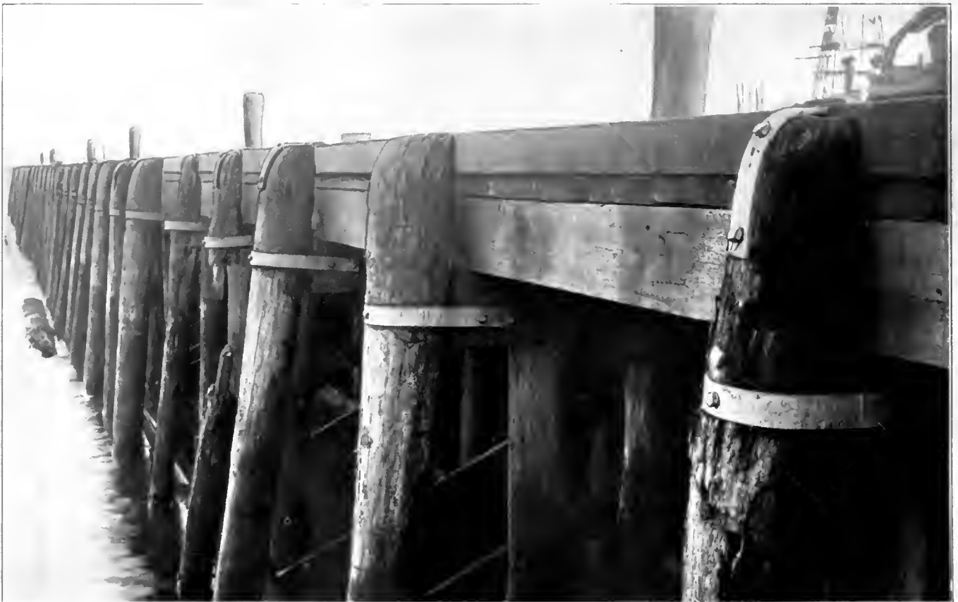
LONGLEAF PINE USED FOR PILING
