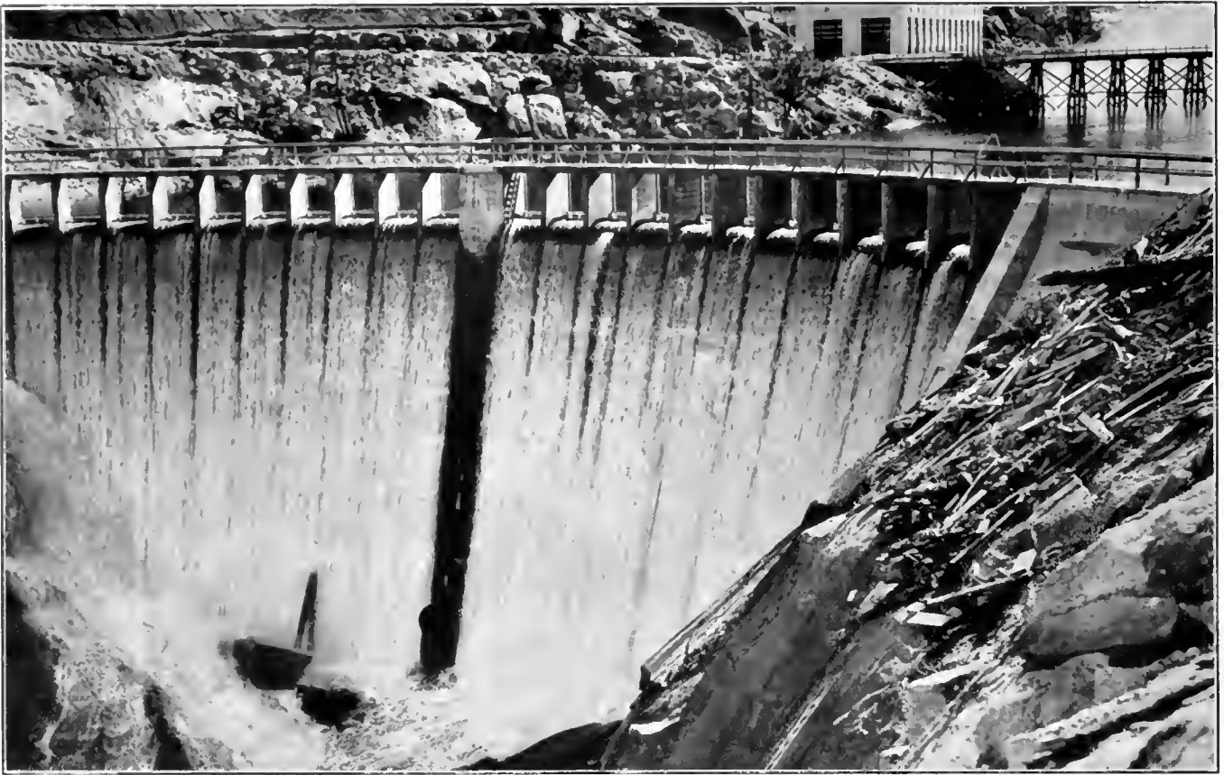
DIVERSION DAM FOR PLANT NO. 2 OF THE PACIFIC LIGHT AND POWER CORPORATION
