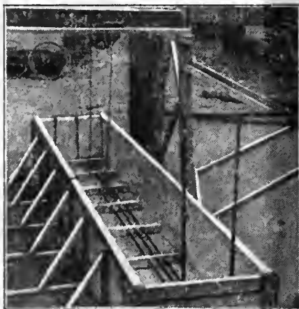
Open-Tank Creosoting-Plant. Note the steam supply-pipes in the foreground and the steam-pipes in bottom of tank arranged in two coils of three lengths each; also the overhead two-ton chain-block traveling-hook.
