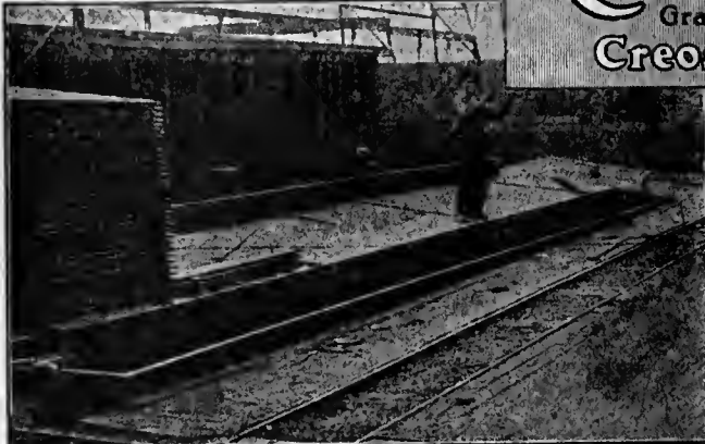
Permanent plant for creosoting of refrigerator-car sills and roof-boards.
