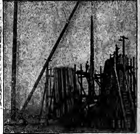
Modern Open-Tank Pole-Treating Plant. (Photo. courtesy Lindley Bros. Co., Minneapolis.)
