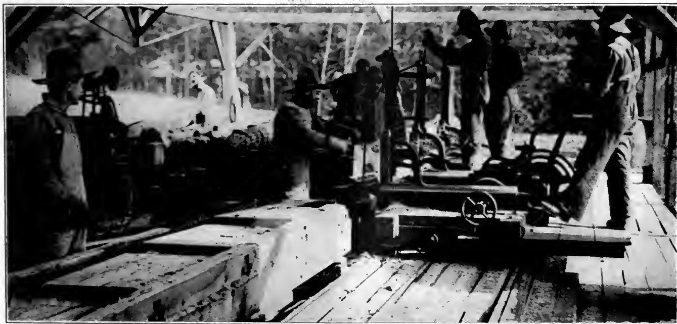
WHERE THE SOUND OF THE SAWMILL BLENDS WITH THE ROAR OF ARTILLERY
