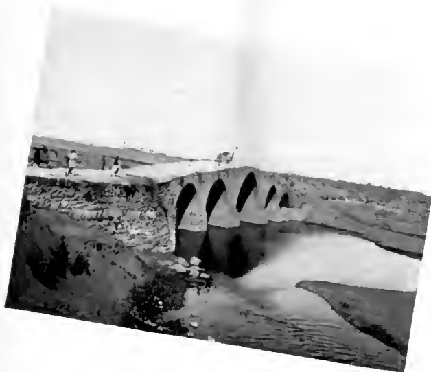
BRIDGE NEAR CHU CHI
