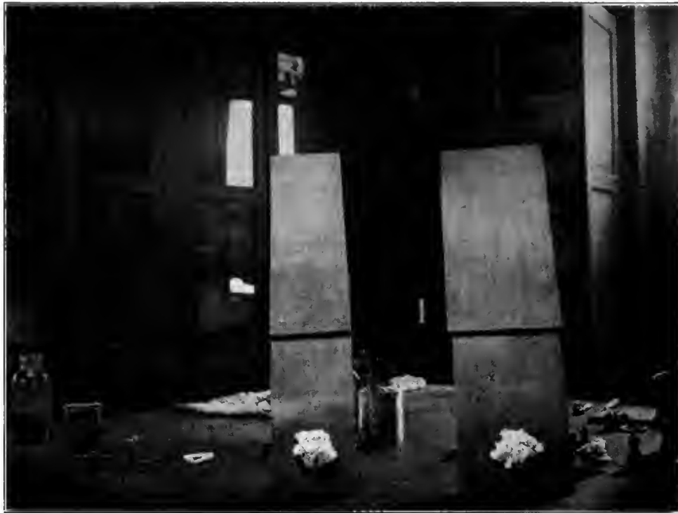
TESTING FIRE RESISTANCE OF SHINGLES
