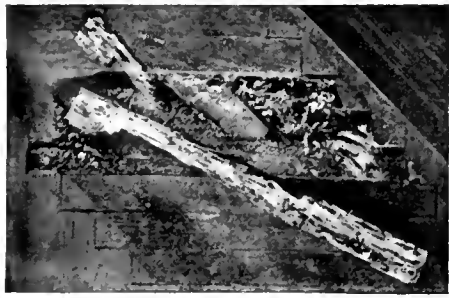
Oak floor honeycombed by white ants (termites). [Reproduced from Farmers' Bulletin 1037, U. S. Department of Agriculture]
