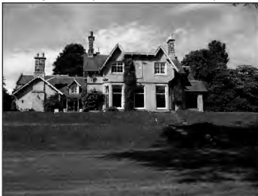
Fig. 5. Rockville house and garden in 2012. The slopes between the terraces were probably rockeries in Fraser's garden.
